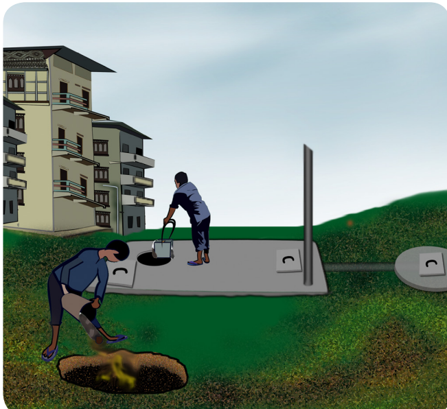
Figure 10. Safe disposal of sludge manually
