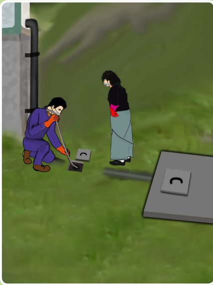
Regularly check pipes and inspection chamber
