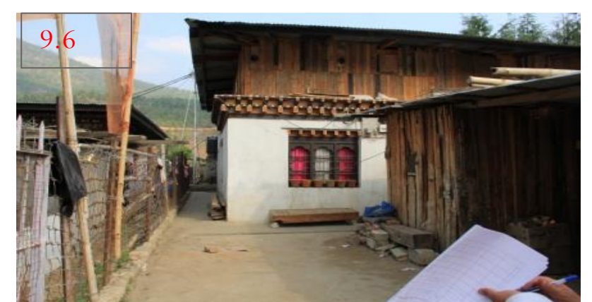
Fig. 9.1: Chang Dungkha clustered village, Fig. 9.2: 3 storied RCC structure, Fig. 9.3: Resort built with RCC, Fig. 9.4: Hotel Holiday Home (single storied RCC structure), Fig. 9.5: DOR office and staff quarters (single storied ekra structures), Fig. 9.6: single storied concrete house with vertically extended wooden attic and Fig. 9.7: new RCC building under construction at the entrance gate of College of Education, Paro.
