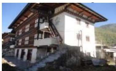
Residential building (Single ownership bungalow type, apartment type, quarters, etc.)
