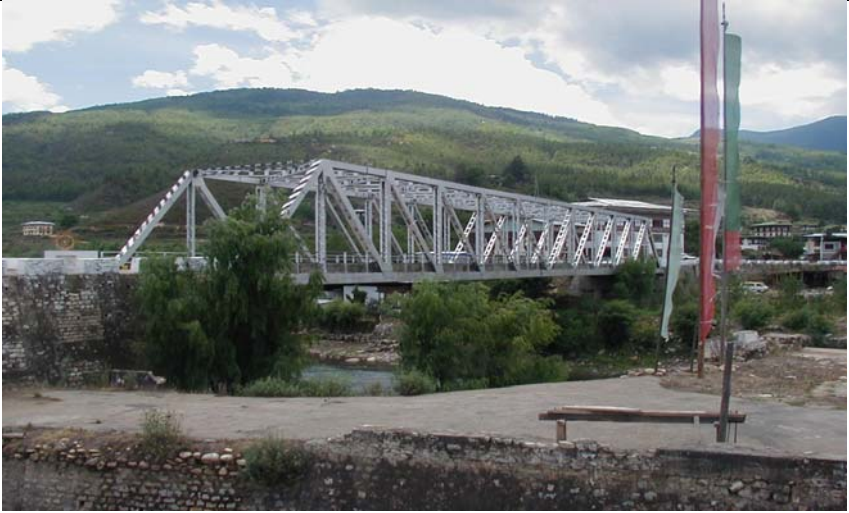
Bondey Zam, (Paro Dzongkhag), Steel Truss Bridge, 67.0 m
