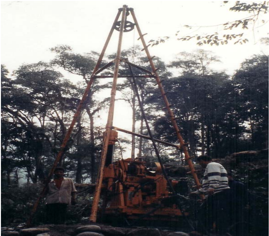
Core Drilling at Bridge Foundations
