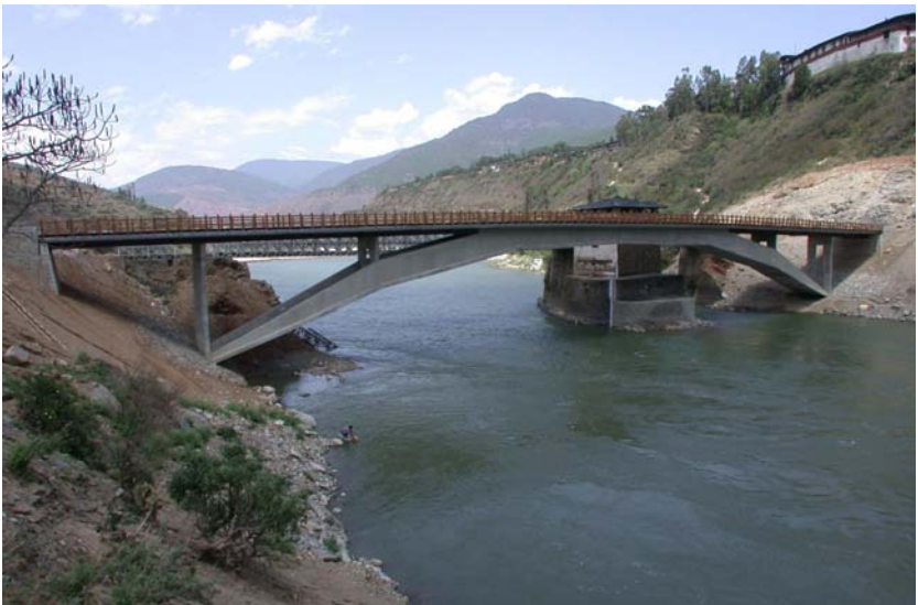
Punatshangchu Bridge (Wangdue), RC Polygonal Arch, Span 120 m
