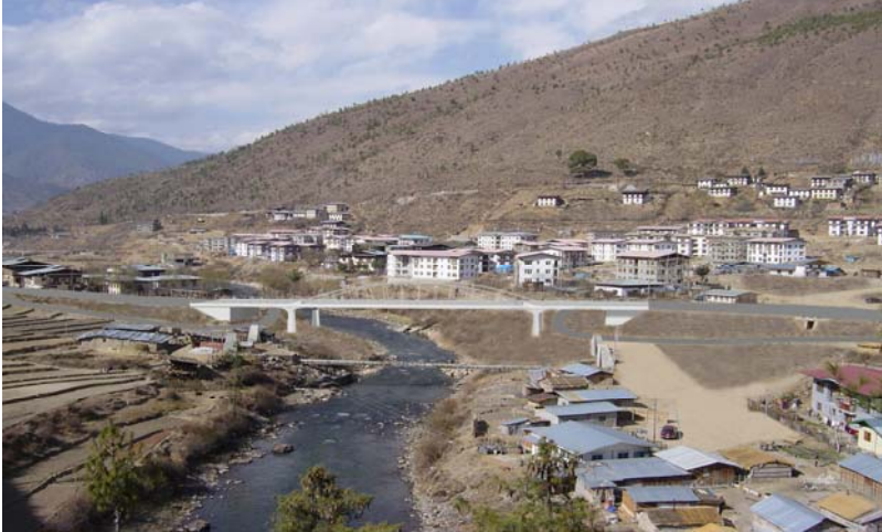
Thimphuchu Bridge (Expressway), Continuous Girder Steel Arch, Span 78.0m
