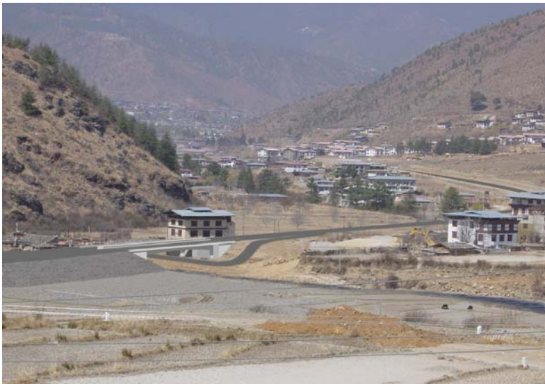
Semtorongchu Bridge (Expressway), Post-tensioned Box Girder, Span 43.5m
