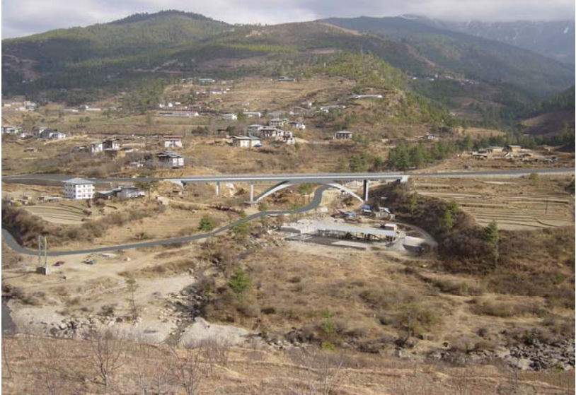
Ngabirongchu Bridge (Expressway), RC T-Girder Arch, Span 123.0 m
