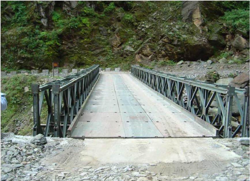
Bailey Bridge with steel decking
