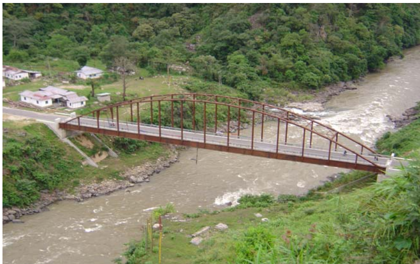
Mangde Zam (Zhemgang Dzongkhag), Steel Langer Arch, Span 95.2 m
