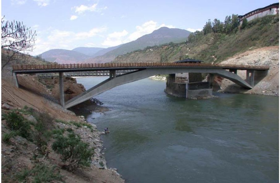
"Bridging the Gaps"
