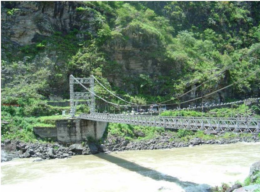
Bailey Suspension Bridge
