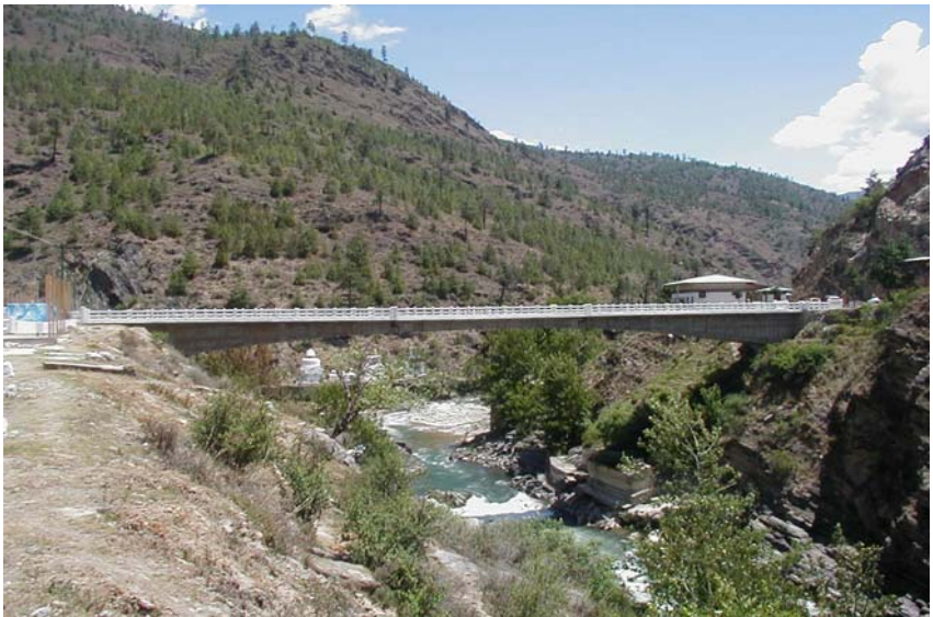
Chunzom Bridge, Prestressed Concrete Cantilever Bridge, Span 77.0 m
