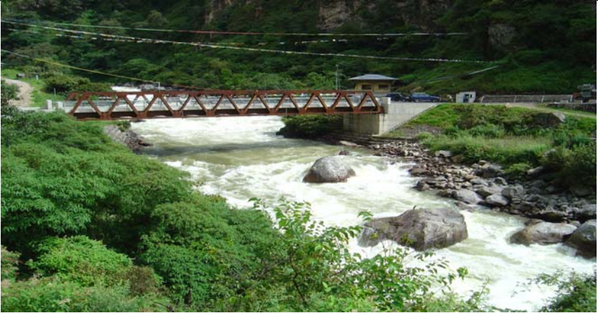
Bjee Zam (Trongsa Dzongkhag), Steel Pony Truss, Span 43.0 m
