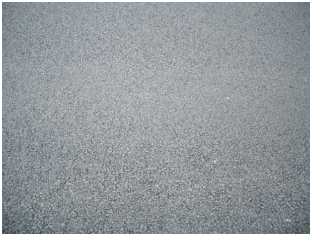
Finished asphalt surface
