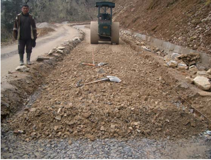
Laying & rolling of sub base layer
