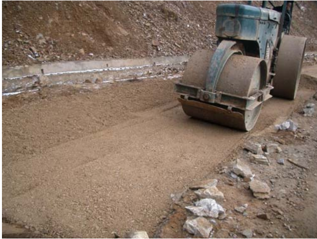
Compaction of base course
