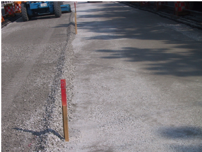
Finished surface of base course
