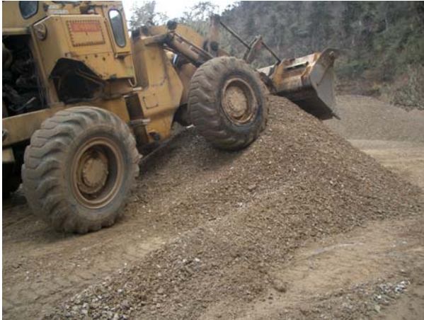
Mixing of materials by machine
