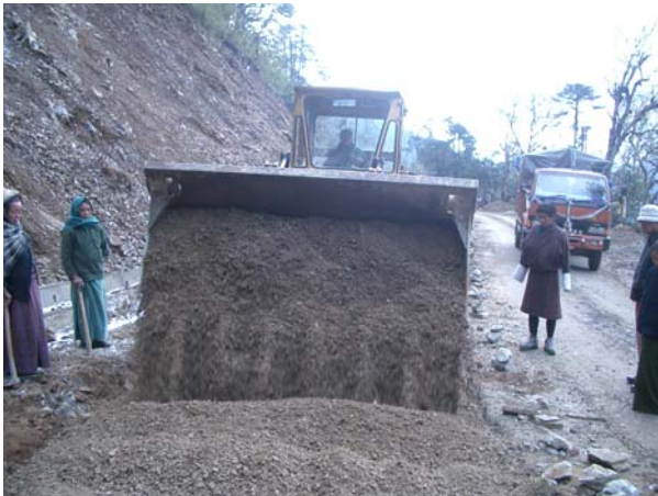
Laying of base course layer
