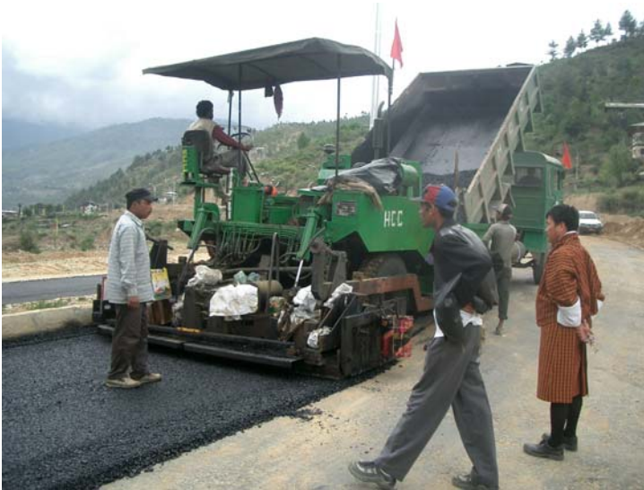
Laying by paver
