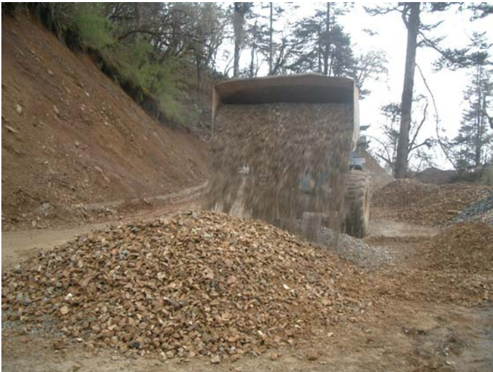
Mixing of sub base material
