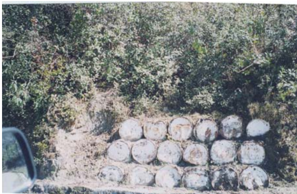
Figure 15: Bitumen Drum Wall
