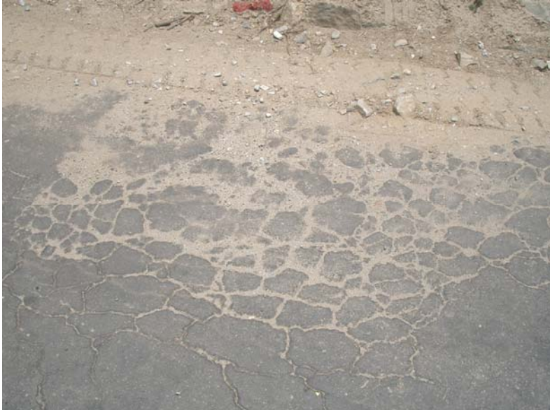
Figure 5: Crocodile Cracks
