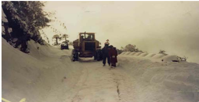
Figure 14: Snow Clearance by machine
