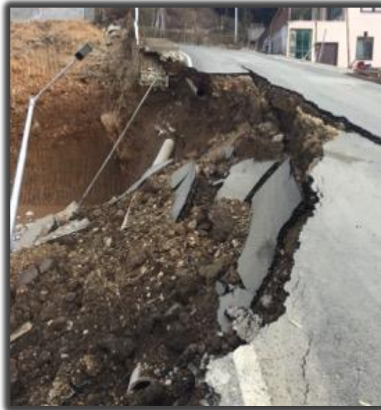
Pictures 1, 2 & 3: Unmonitored developments on very steep slope leading to infrastructure and environmental damage
