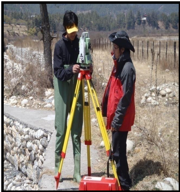
Figure 13: Setting out Total Station
