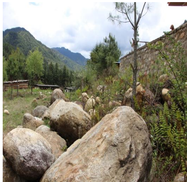
Figure 4: Boulders deposited at Choekhor Toe PS ground by 2009 flood.
