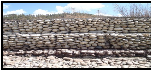
Figure 15: Gabion wall for flood protection on the upstream of airport.
