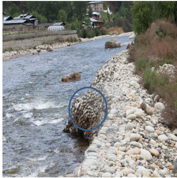
Figure 5: Chamkhar Chu right bank below Wangdicholing Figure 6: Bulged gabion wall below Wangdicholing
