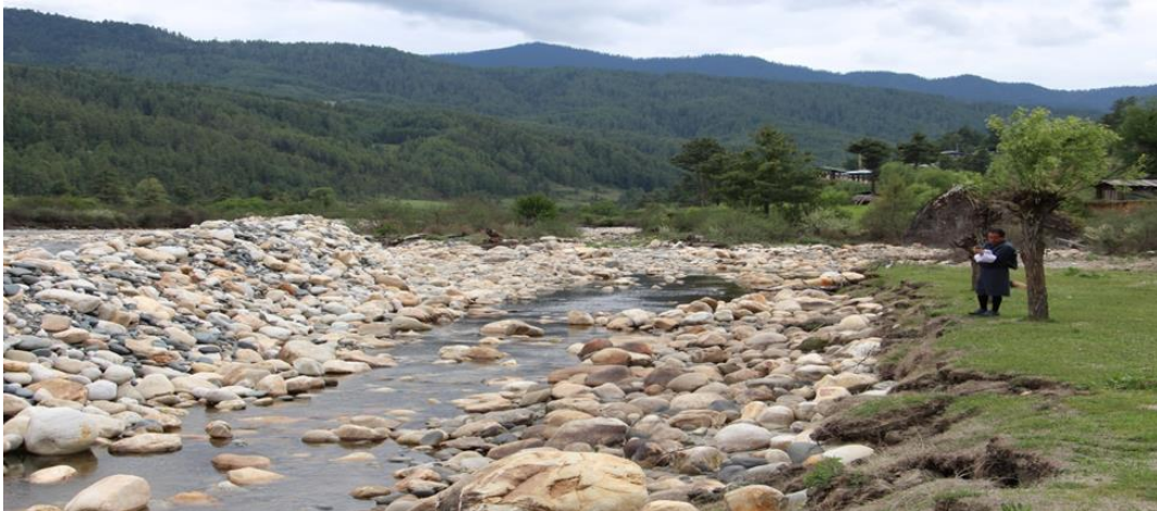
Figure 11: Dredging works at Nimalung Ju
