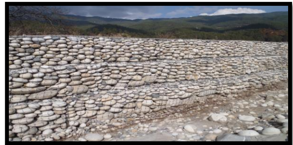
Figure 16: Gabion wall for flood protection on the downstream of airport.
