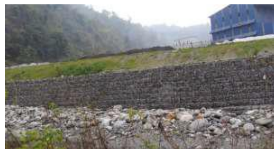
Figure 30: Flood Protection Works along Barsa chu.
