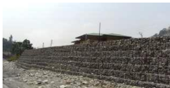
Figure 29: Flood Protection Works along Barsa chu.
