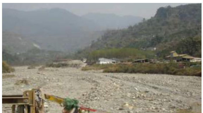
Figure 28: Balujora river posing threat to the BBPL factory at Pasakha.
