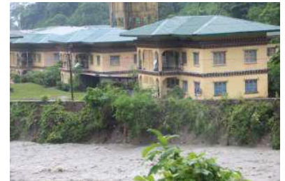
Figure 7: The flood protection structure protecting the housing colony.
