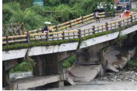
Figure 9: The Bhalujhora Bridge.
