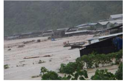
Figure 4: Damages caused by Amochu.
