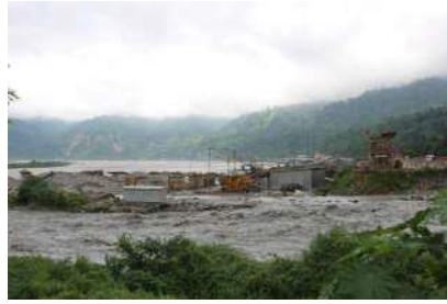
Figure 3: Damaged caused to the properties at the confluence of Dhoti Khola.
