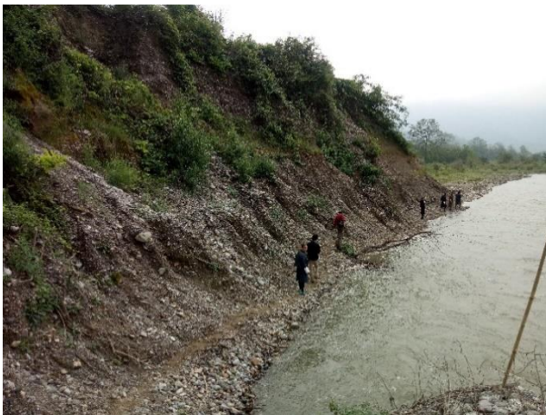
Figure 17: Scouring/Erosion by Sunkosh River at the base of Kalikhola
