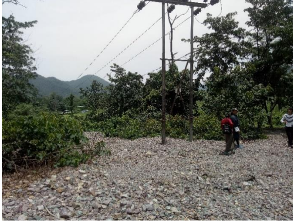
Figure 19: Debris from Pairini stream affecting the electric pole in Karmaling village
