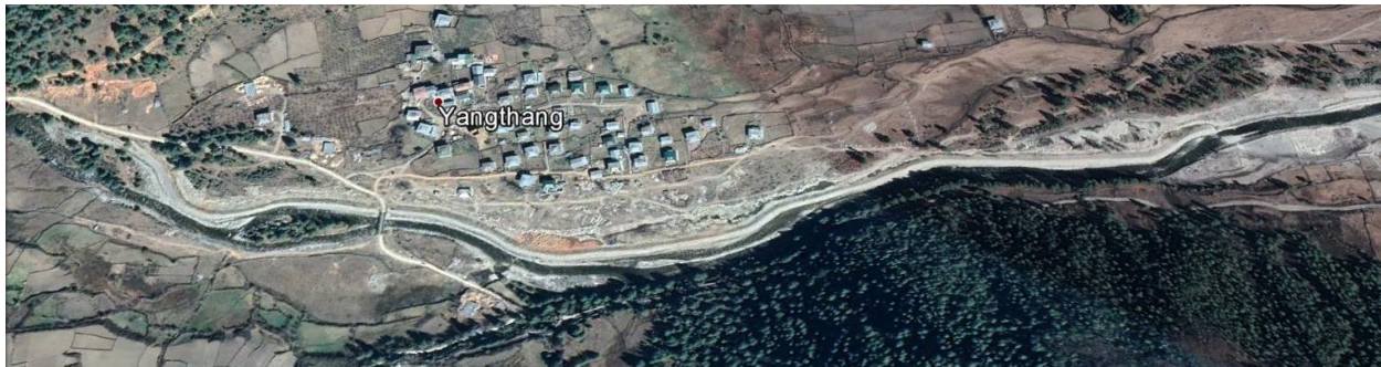
Figure 27: Haa River along Yangthang Village in Haa Dzongkhag in year 2016 after constructing gabion revetment to protect the nearby settlements.
