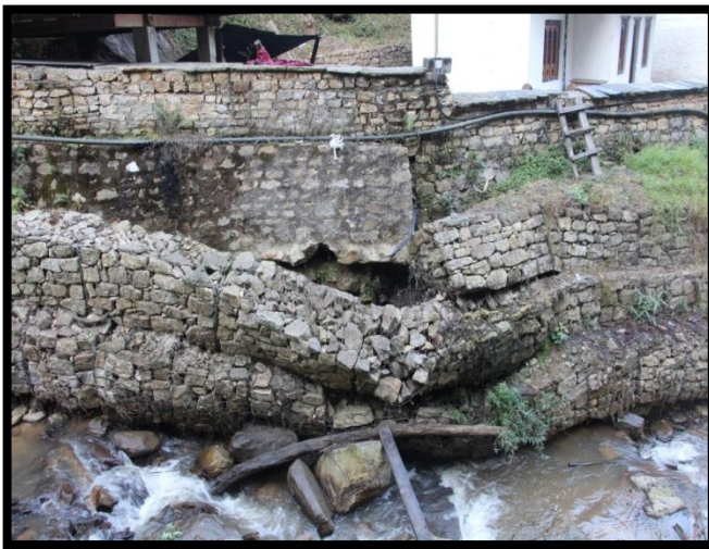
Figure 9: Partially washed away gabion wall at upstream
