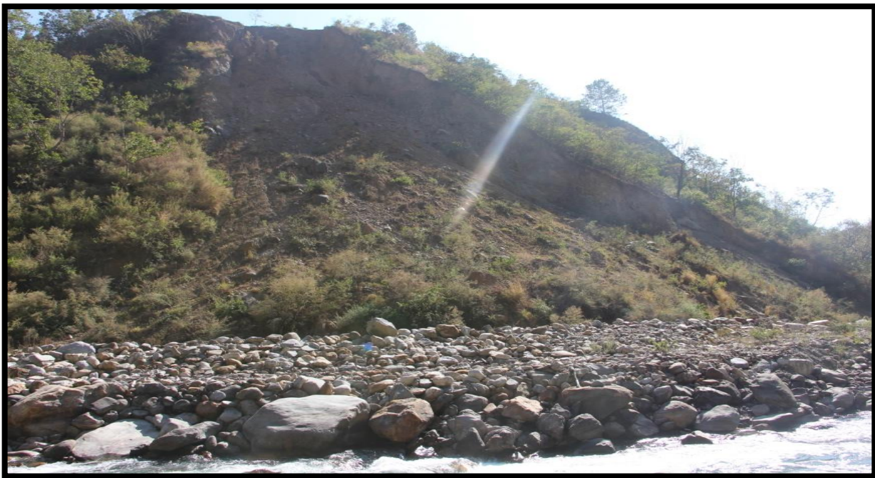
Figure 12: Souring creates landslide below the khoma L.S School.
