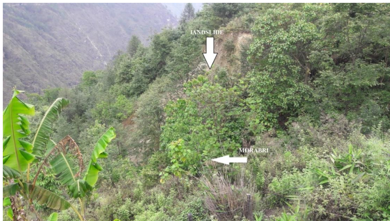
Figure 17: Landslide area along Morabri.
