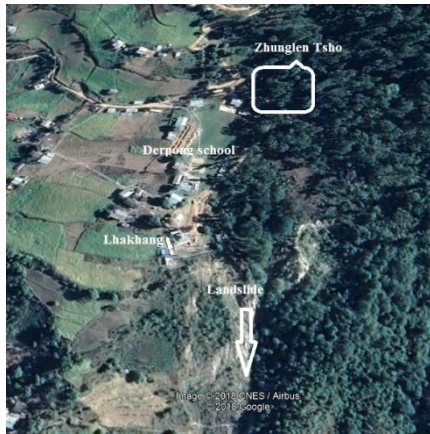
Figure 18: Landslide area below Zhunglen Tsho
