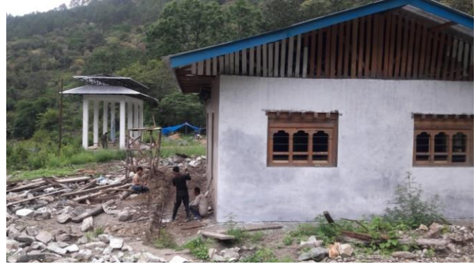
Figure 5: Crematorium under construction
