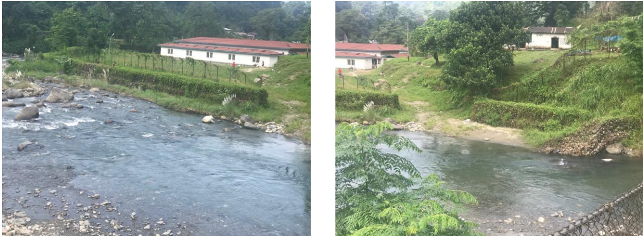
Figure 3: Armed force colony at the right bank of Kerong river and is under risk of inundations during monsoons.
