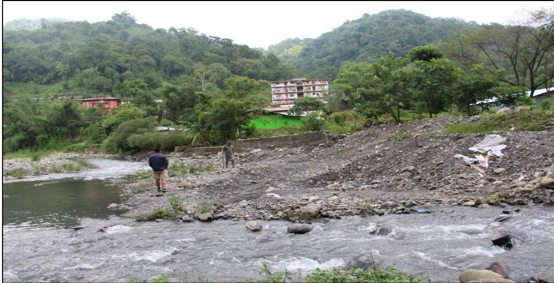
Figure 5: Near DoR office area
