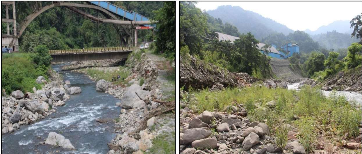
Figure 6: Kerong river flowing adjacent to DCCL area and boulders stacked along the river
