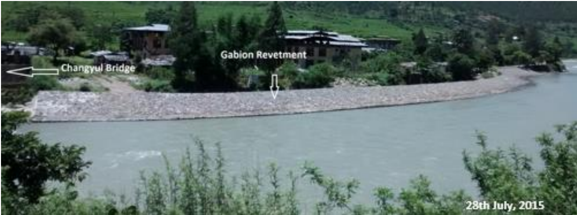
Figure 30: Upstream of Changyul Bridge after construction of Gabion Revetment in 2014
