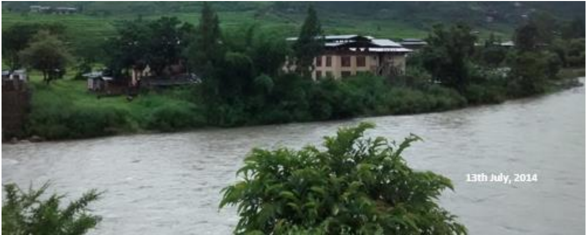
Figure 29: Upstream of Changyul Bridge before construction of Gabion Revetment in 2014
