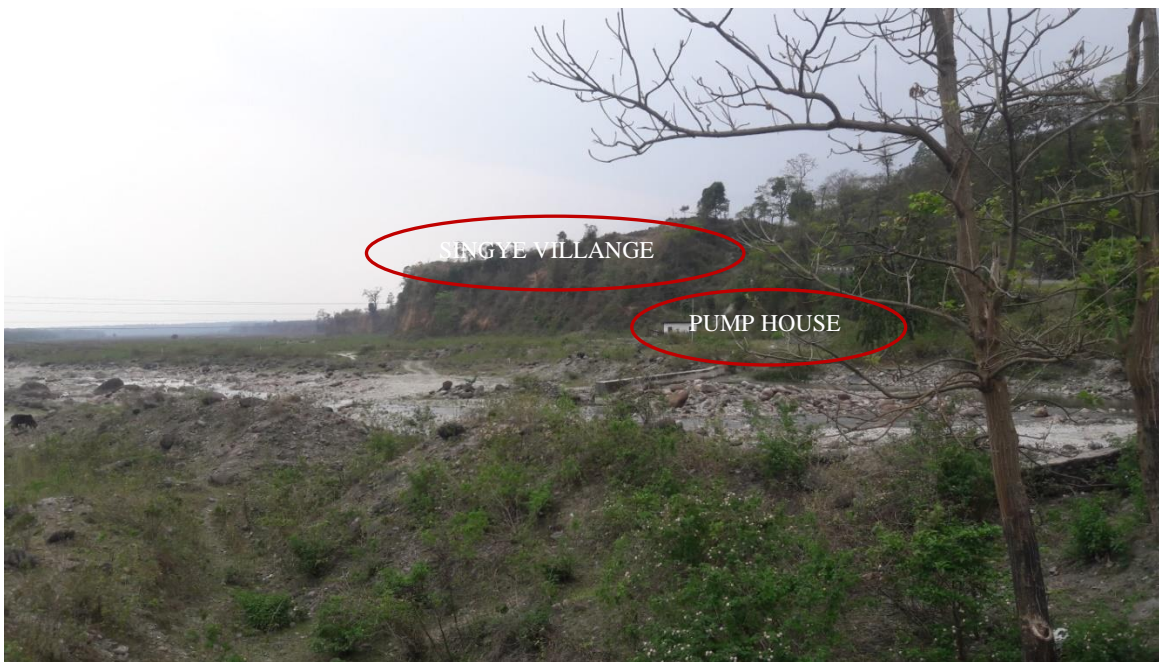
Figure 21: Image of Singye village and pump station along Jiti Khola
