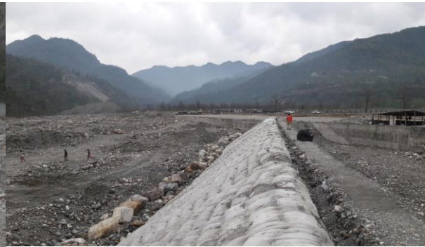
Figure 8: AB Mattress under construction for diversion of Dhamdum river to Budeney river flowpath
