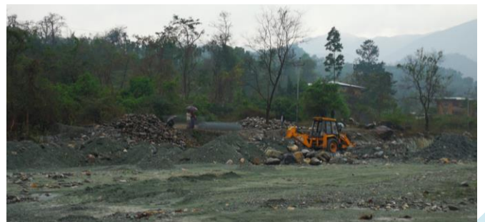
Figure 6: Ongoing flood protection works carried out by DoR
