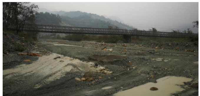
Figure 5: Budney Riverbed filled with heavy sediment deposits
