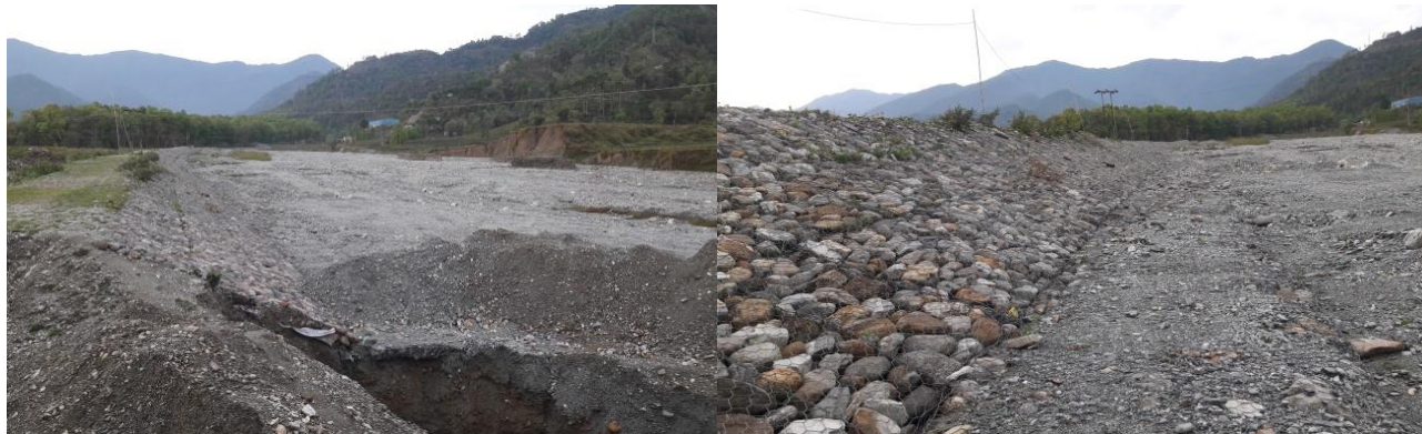
Figure 34: Embankment with gabion crate revetment at right bank along Sukreti River.
