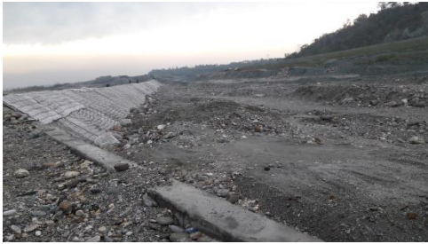
Figure 35: AB mattress construction along Dhamdum River
