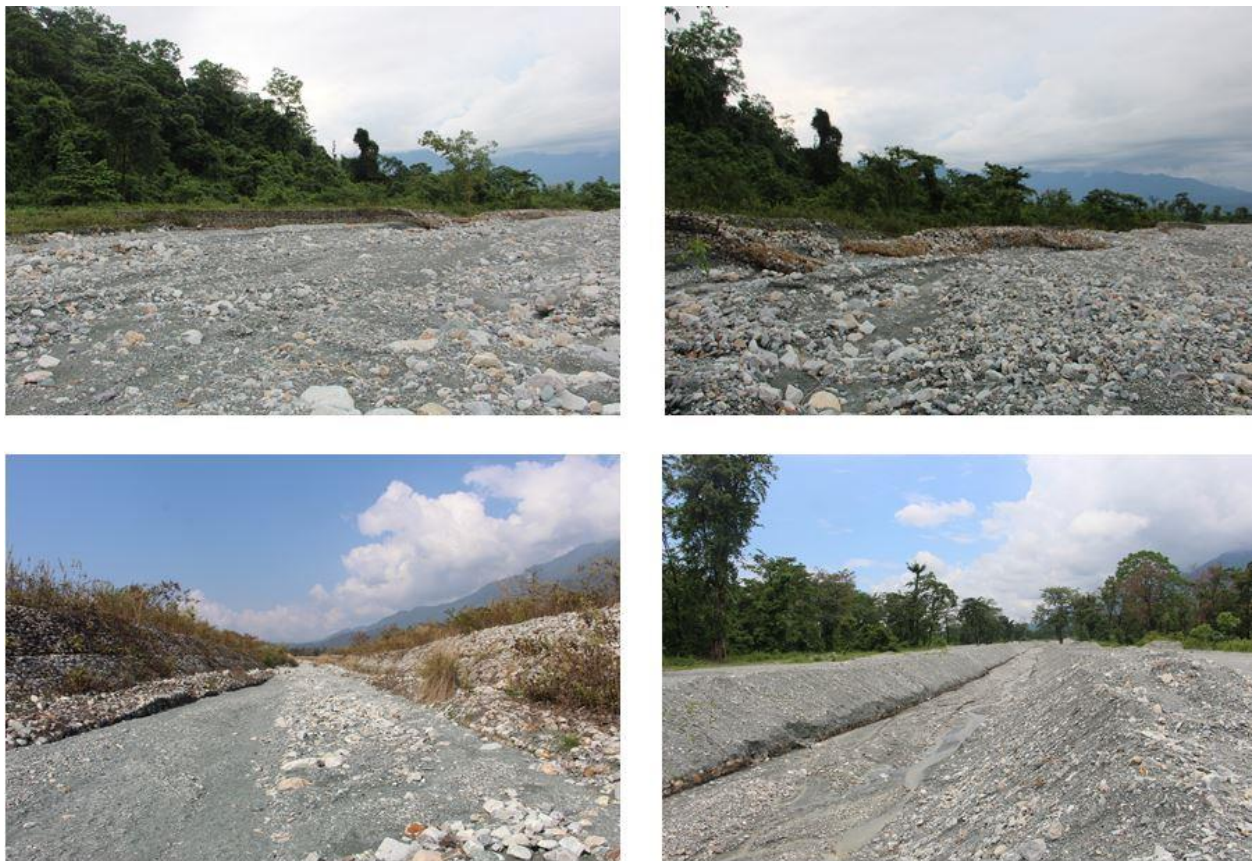
Figure 16: Past interventions along Shetikheri (Gabion walls and floodways).
