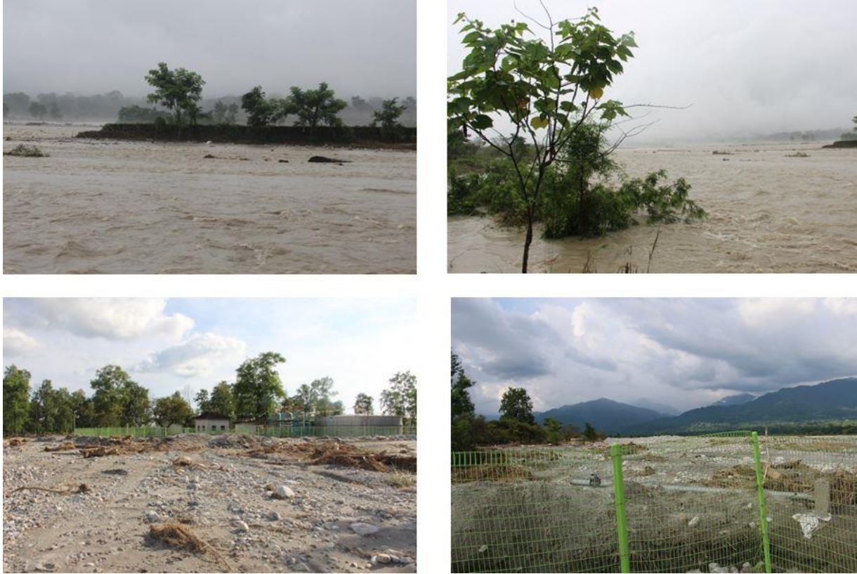
Figure 27: Destructions caused by Mao River near the Infiltration gallery.
