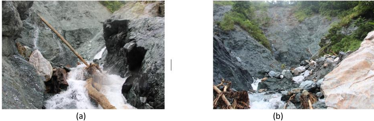
Figure 14: (a) Source of Shetikheri (b) Landslide at source.
