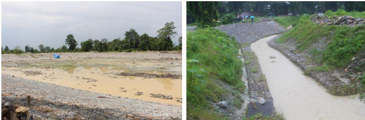
Figure 12: Detention pond and floodway in Gelephu.
