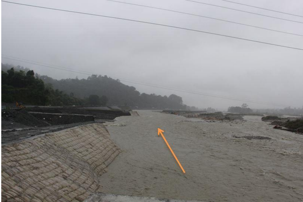
Figure 25: Sarpang Chhu changed its course towards the left bank (During Flood).
