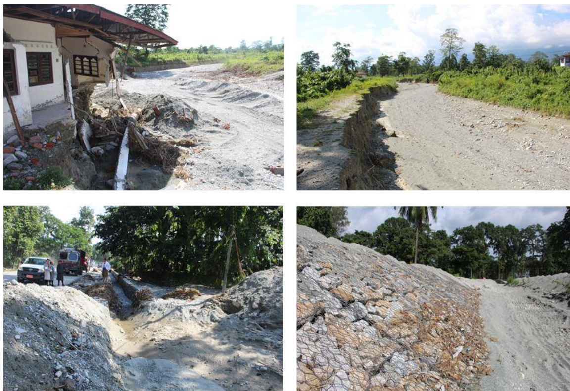
Figure 41: Flood damages along small Aipoly.
