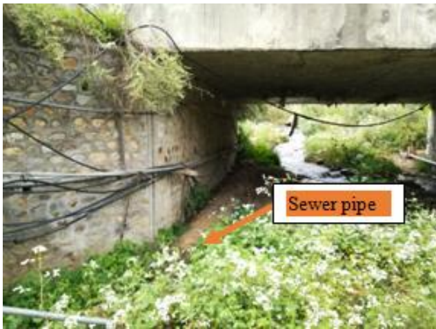
Figure 26: Sewer pipe laid on the stream bed below Chubachu Zam
