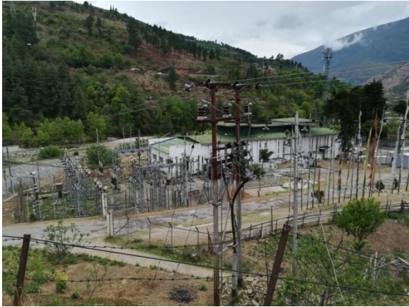
Figure 42: Area near the Begana Mini Hydel project
