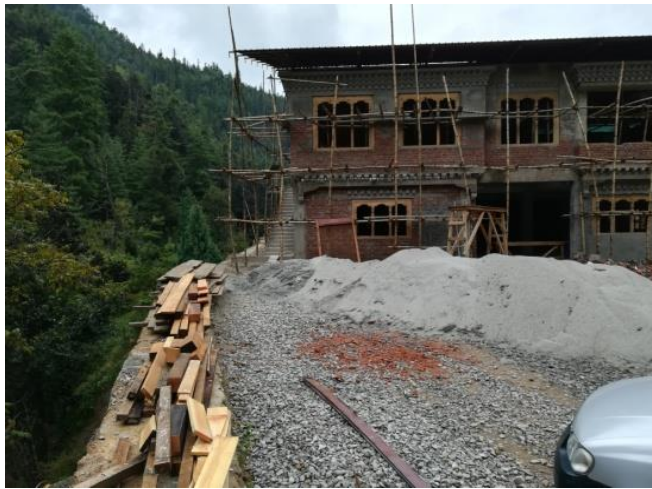
Figure 33: Living water company infrastructure under construction (October, 2017)
