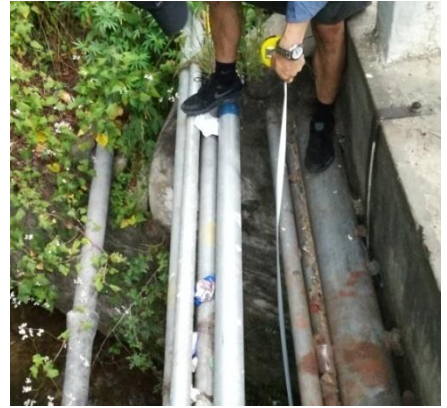
Figure 29: Water Pipes laid at the same level as Desi Zam
