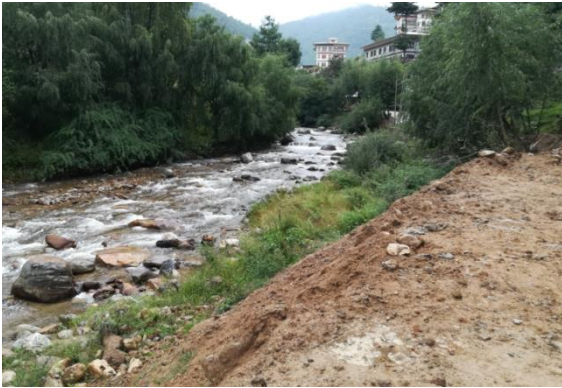
Figure 35: Need for a retaining wall upstream of Semtokha Bridge
