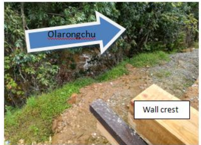
Figure 34: The distance between retaining wall crest and Olarongchu
