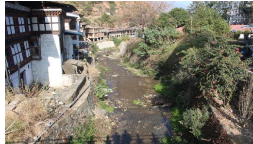
Figure 4: RRM wall at both banks.
