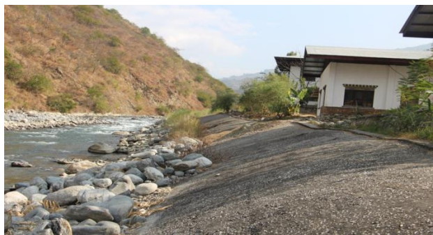
Figure 8: PCC revetment along Rangjung TTI
