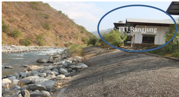
Figure 31: Embankment with PCC revetment along Gamri Chu in Rangjung.
