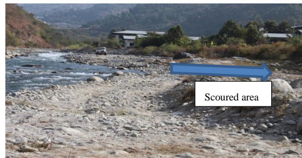
Figure 7: Scoured area downstream of TTI, Rangjung.
