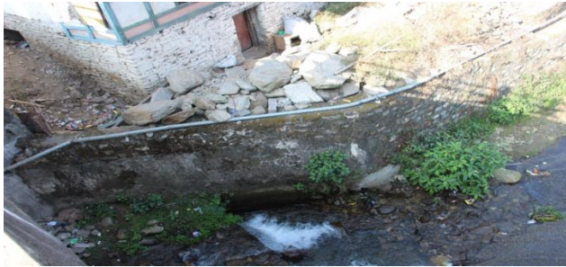
Figure 3: Downstream of highway bridge
