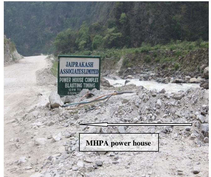
Figure 6. Location of MHPA powerhouse.
