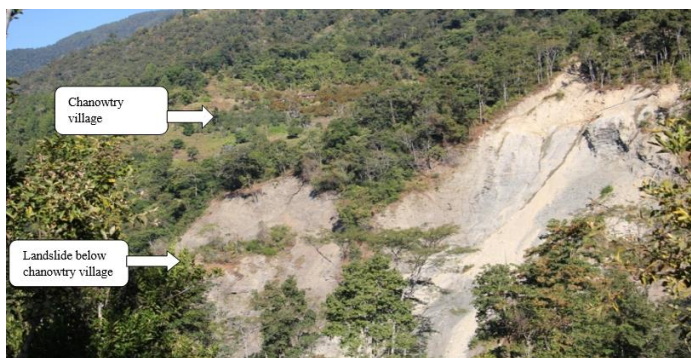
Figure 5: landslide area in Lower chanowtry village .
