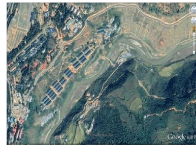
Figure 11: Temporary sheds of Labours in Wangdue Dzong reconstruction project under threat.
