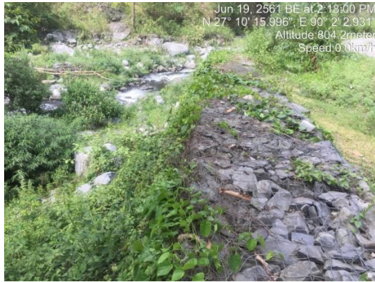
Figure 4: Gabion wall constructed by PHPA II along Kamichu
