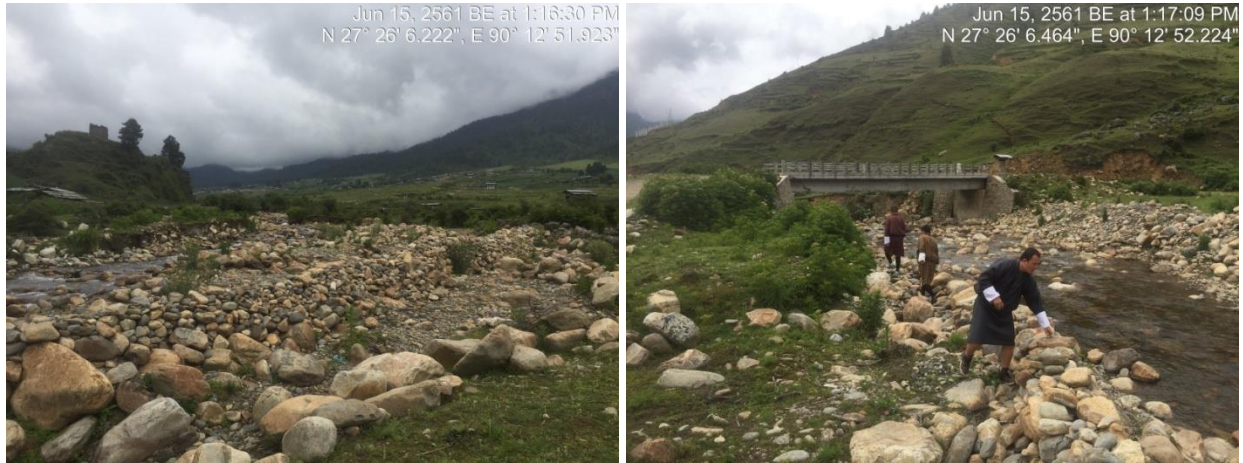
Figure 19: Upstream of PakshingZangpa bridge.
