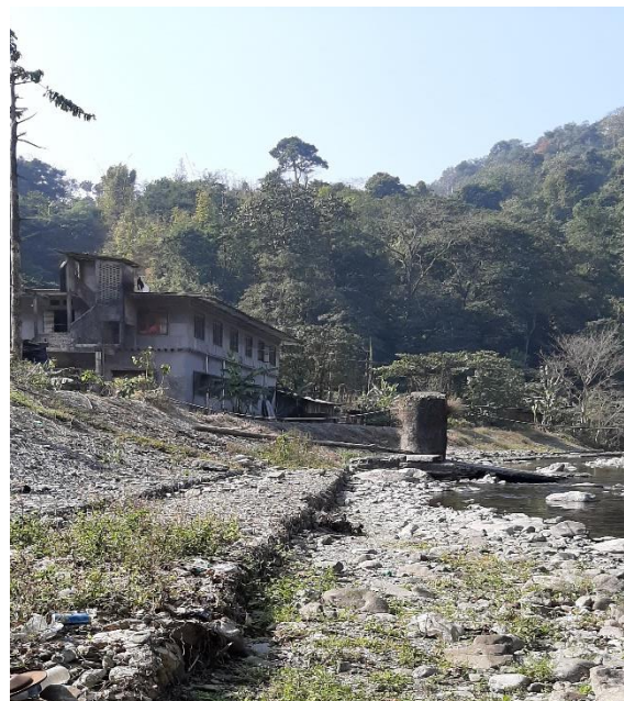
Figure 22 Gabion revetment below the motorable bridge
