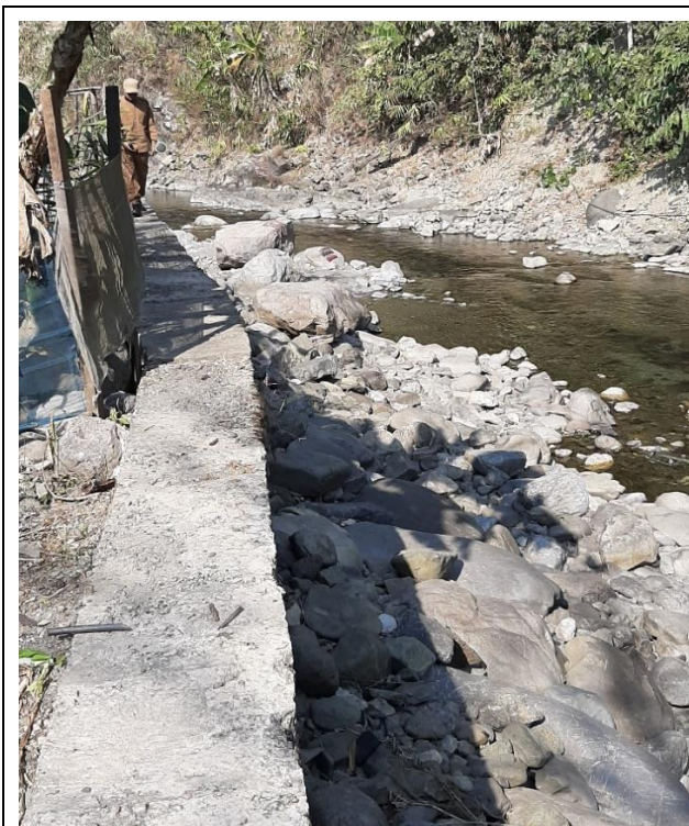
Figure 26 Existing RCC structures
