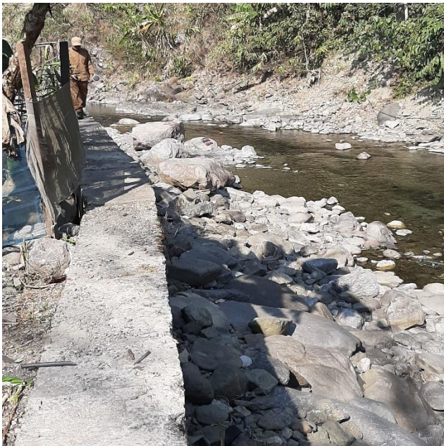
Figure 21 RCC wall near the automobile workshop
