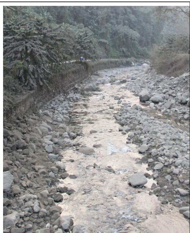
Figure 27 Existing gabion wall
