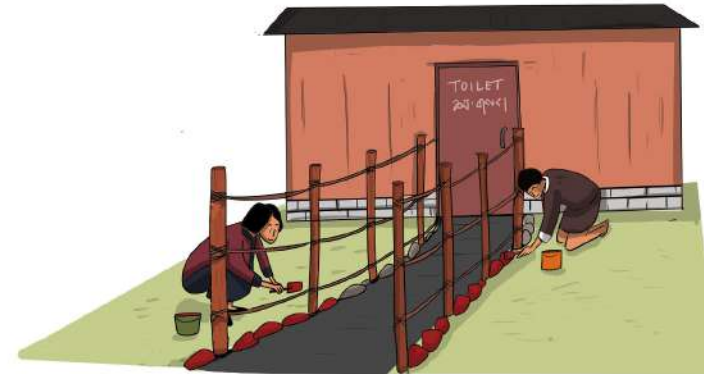
Figure 6: Alternatively use guiding rope with no obstructions for persons with vision impairment. The height of the guiding rope should be 2ft 6 inches – 3 ft) above the ground. Consider provision of white cane/stick
