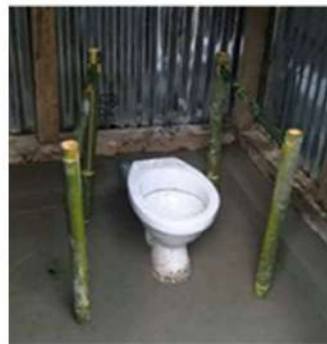
Figure 1: Use European pot (sitting) instead of the Indian ceramic pan. Install/fix grab bars and rails on the floor/wall (Grab bar height should not be more than 2 ft 6 inches).
