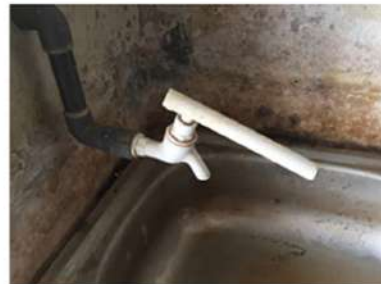
Figure 3: Install long tap handles or modified (with long plastic handles) to make easier to turn. Consider use pedal/foot control as per the needs of the household members
