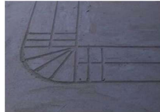
Figure 6: Tactile markings etched to alert to users (vision impaired) when getting to and approaching toilet pans
