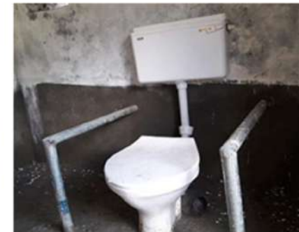
Figure 1: Use European pot (sitting) instead of the Indian ceramic pan. Install/fix grab bars and rails on the floor/wall (Grab bar height should not be more than 2 ft 6 inches).
