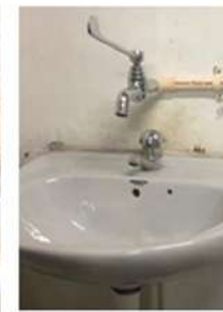
Figure 3: Install long tap handles or modified (with long plastic handles) to make easier to turn. Consider use pedal/foot control as per the needs of the household members
