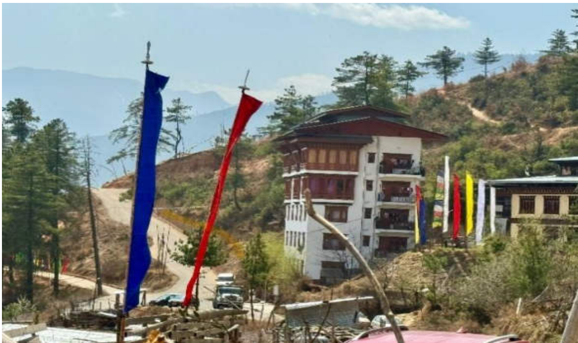
Image 2: Realignment of trunk line pipe section due to possible slope instability below lhakhang steep gradient
