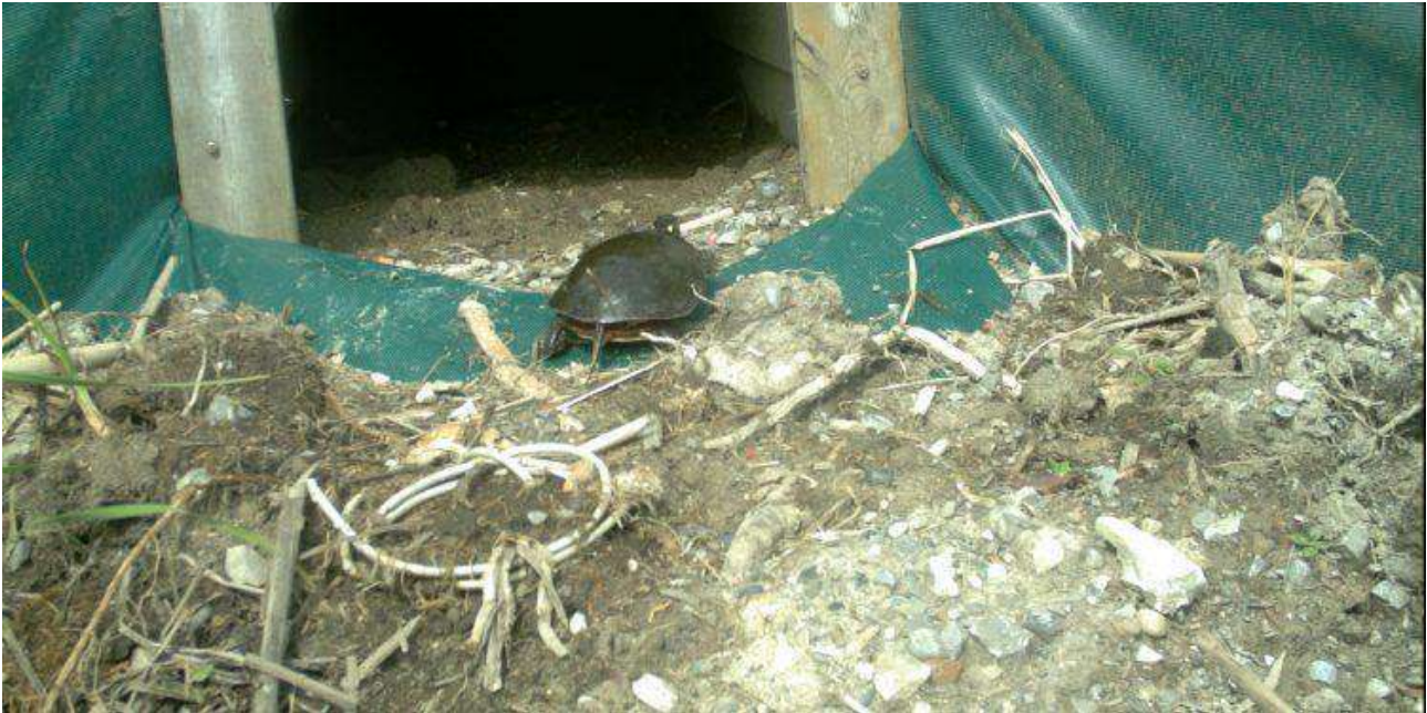
Figure 10.3 A Midland Painted turtle enters one of the new culverts that were installed under the Causeway in the fall of 2014 to enable wildlife to pass safely under the busy road 56
