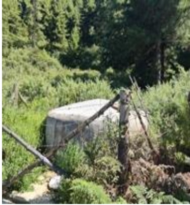
Pic-7: Reservoir tank that is climate resilient in terms of design and construction quality
