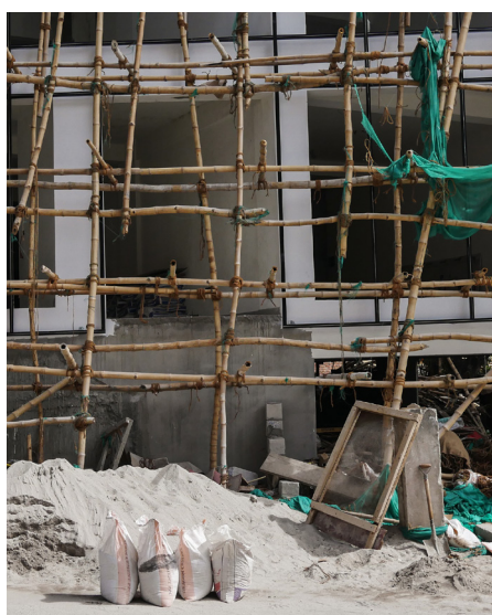
Fig. 3.7 (left): Raw bamboo poles used as scaffolding © Kéan Koschany, 2024
