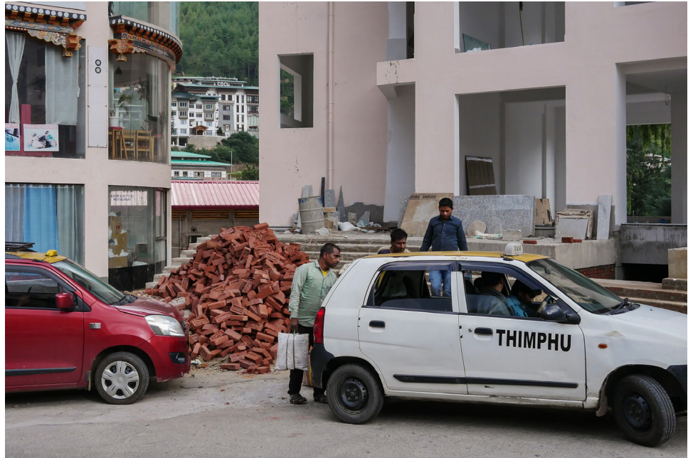
Fig. 3.40: Migrant construction workers in Thimphu © Kéan Koschany, 2024
