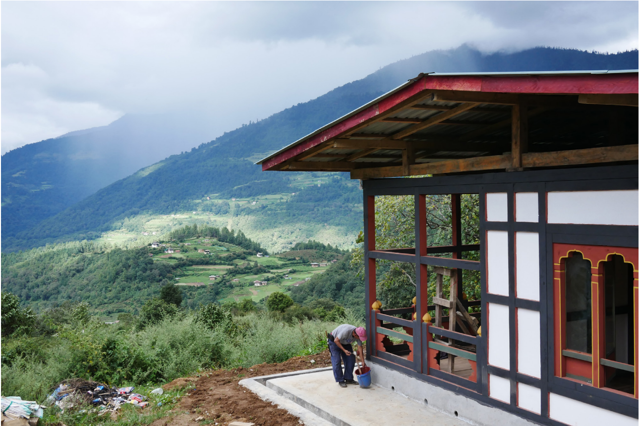
Fig. 3.36: Local artisan painting the timber structure of a new building © Kéan Koschany, 2024
