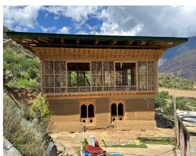
Fig. 3.20: Rural building utilising rammed earth, bamboo, and hempcrete in Gomche, Paro © Matěj Vacek, 2025
