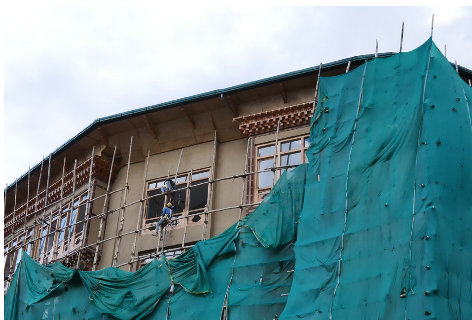
Fig. 3.28: Construction workers on a scaffolding at a construction site in Thimphu © Kéan Koschany, 2024
