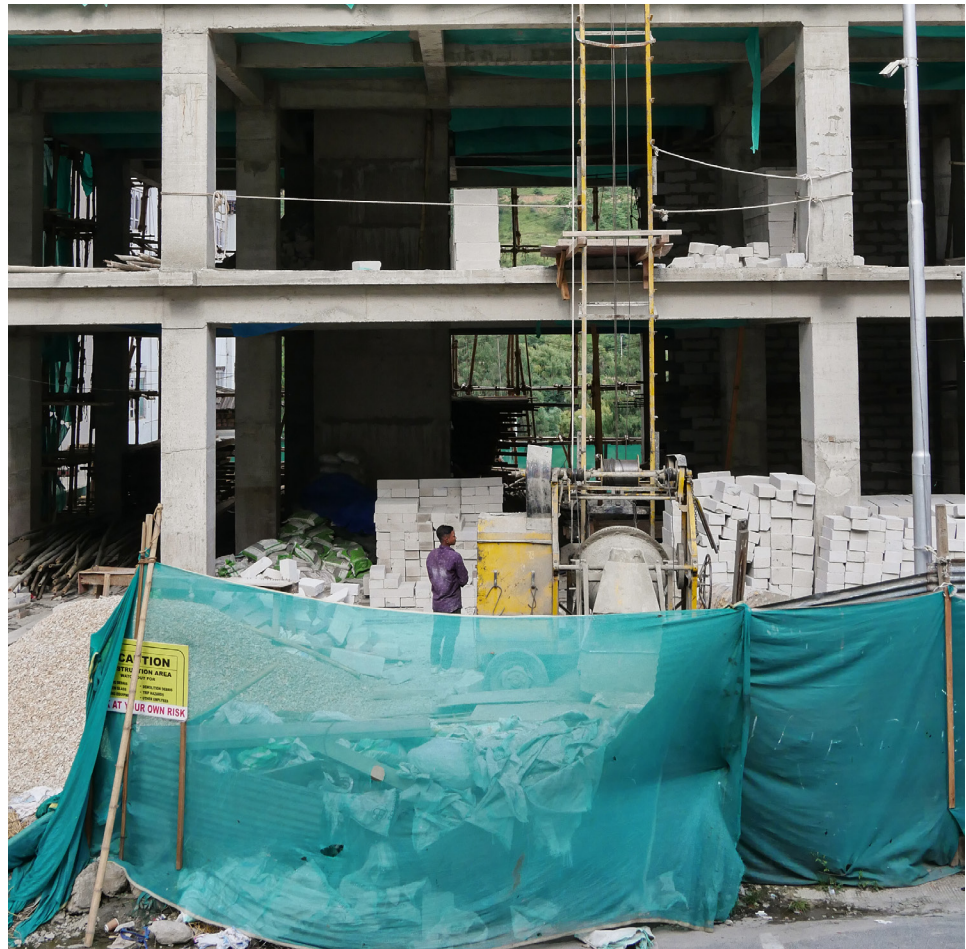
Fig. 2.2: Construction site of a RCC frame building in Thimphu ©Kéan Koschany, 2024
